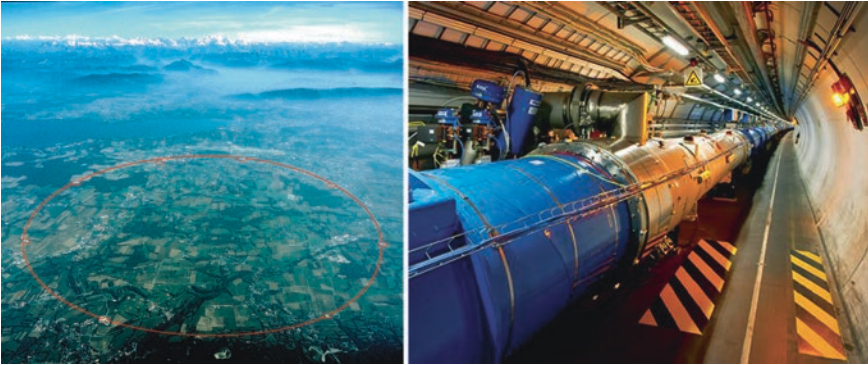
Fig. 14.1 The Large Hadron Collider (LHC) in Geneva Switzerland lies underground in a circular tunnel with a circumference of nearly 30 km. It is the largest particle accelerator in the world. The LHC achieves energies of E = 14 TeV, which correspond to temperatures of T = 10^{17} K and a time of t = 10^{-14} s after the big bang Credit CERN
