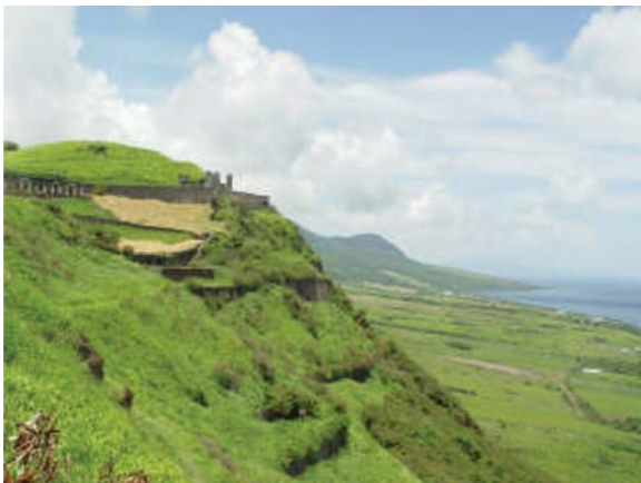
Fig. 5 Brimstone Hill, British hillside fortification, St. Kitts (photograph by D. Armstrong)
