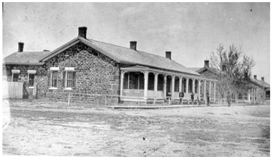
Fig. 1 The officers' quarters at Fort Larned, Kansas, exemplify the higher status that officers of the frontier Army enjoyed (Fort Larned National Historic Site photograph)
