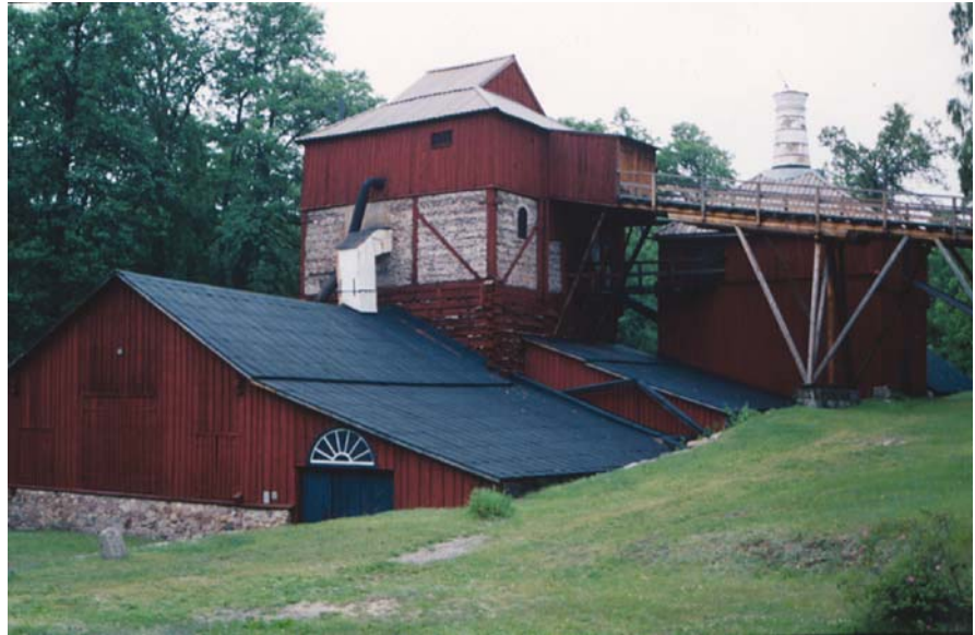
Fig. 2 The eighteenth-century Englesbergs Bruk blast furnace iron-making complex, Norberg, Sweden, which is listed as a World Heritage Site (photograph by the author)
