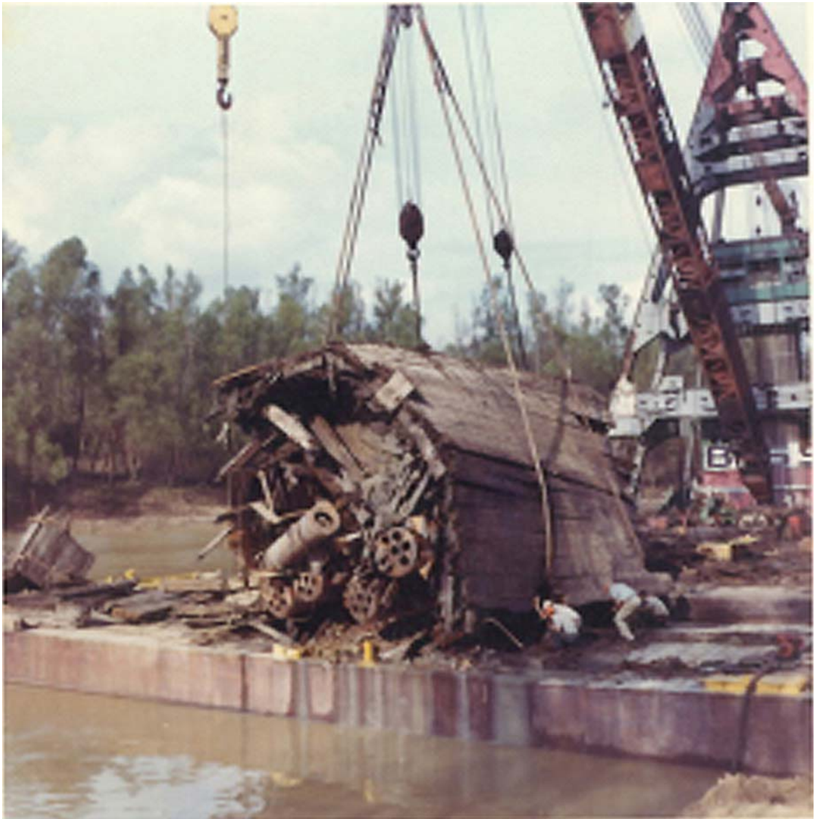
Fig. 14 Attempts to raise the USS Cairo from the bottom of the Yazoo River were disastrous (courtesy Vicksburg National Military Park, USDI National Park Service)
